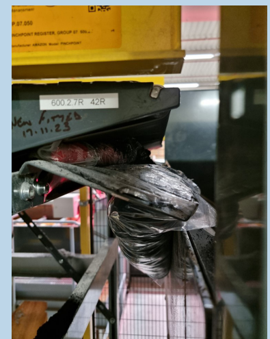
Visible Inspection of Guard
